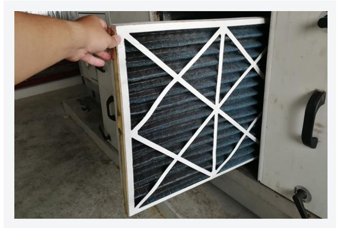
Dirty air filters increase energy consumption, reduce air flow, and expose occupants to harmful particles. Filters should be monitored regularly.
